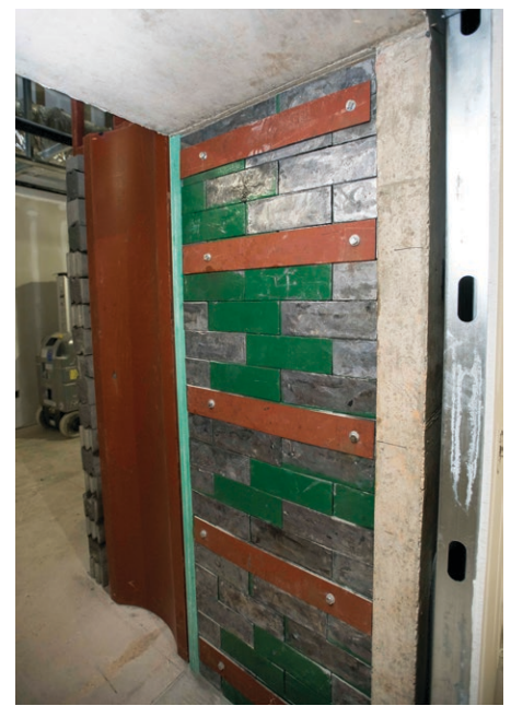
Above: A wall of lead bricks that weigh 40 pounds each were used to add a another layer of protection against escaping radiation from the linear accelerator. Left: A corner infusion room will have a window that will overlook a park area.
