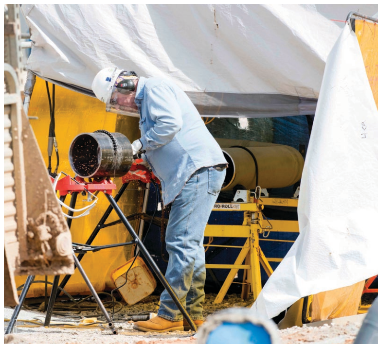
A worker prepares a section of pipe to be welded into the system.
