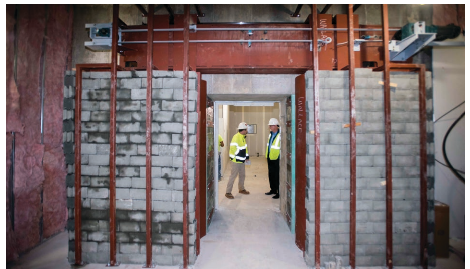
Shelco Project superintendent Jim McKeon talks with Rick Parker, executive director of Novant Health Rowan Medical Center Foundation, inside the LINAC room that will house the new linear accelerator. Behind the special super dense, metal-infused blocks that weigh 50 pounds each is a 15-ton sliding door.
