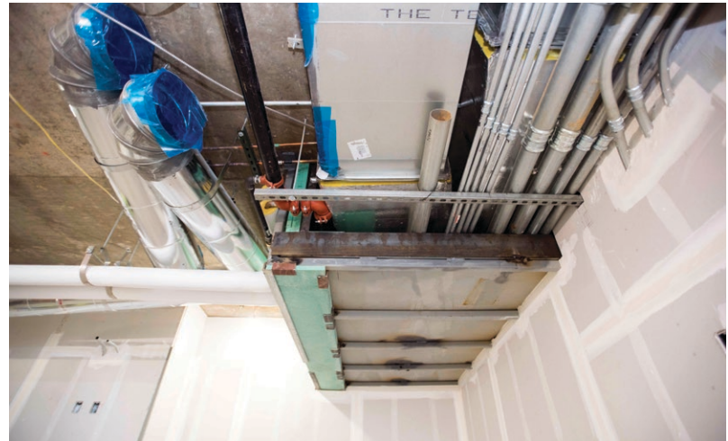
The HVAC and electrical lines inside the linear accelerator room.
