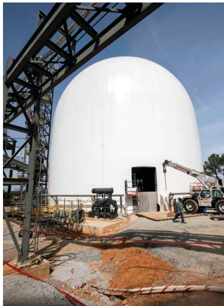
A large domed building will keep the recycled coal ash after compacting before it's off-loaded to be repurposed. The building is ringed by piping that will keep the ash moving and not settled at the bottom.
