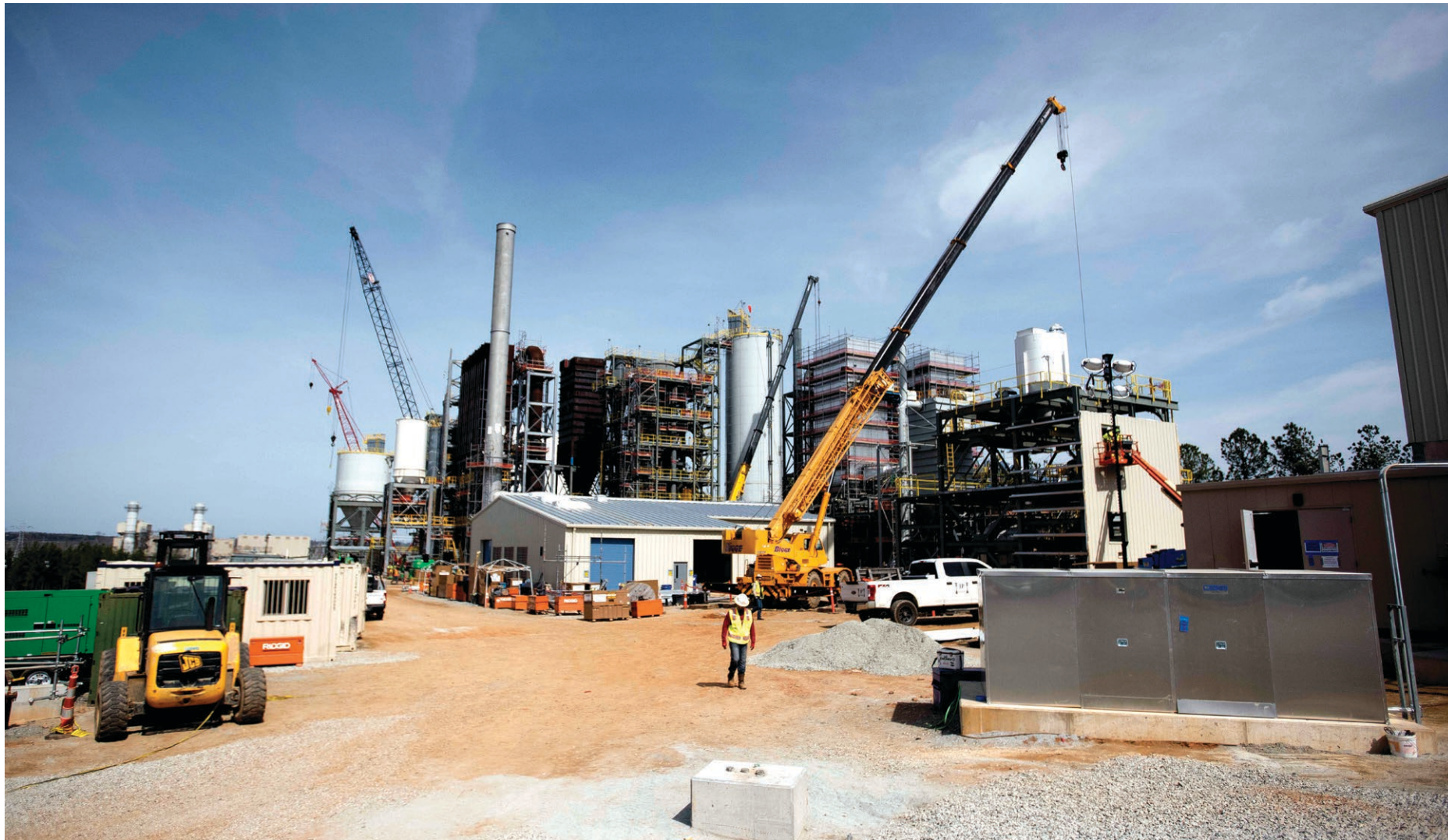
Several cranes and lifts circle the new facility that is being built at Duke Energy's Buck site. Construction continues on a Duke Energy facility near the Buck Combined Cycle plant on Dukeville Road. The new construction is a processing plant that will take spent coal ash from the nearby holding basins and recycle the material. (Jon C. Lakey photos)
