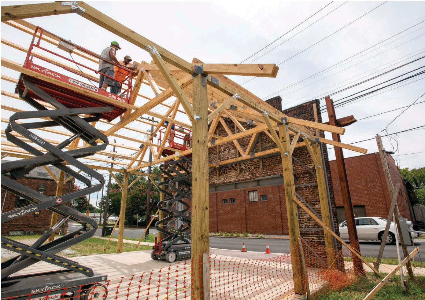
Kevin Moore and Shaun Freeman from R & L Glover Enterprises use a lift to reach the trusses that are installed in the framing out process during construction of the Railwalk Pavilion.
